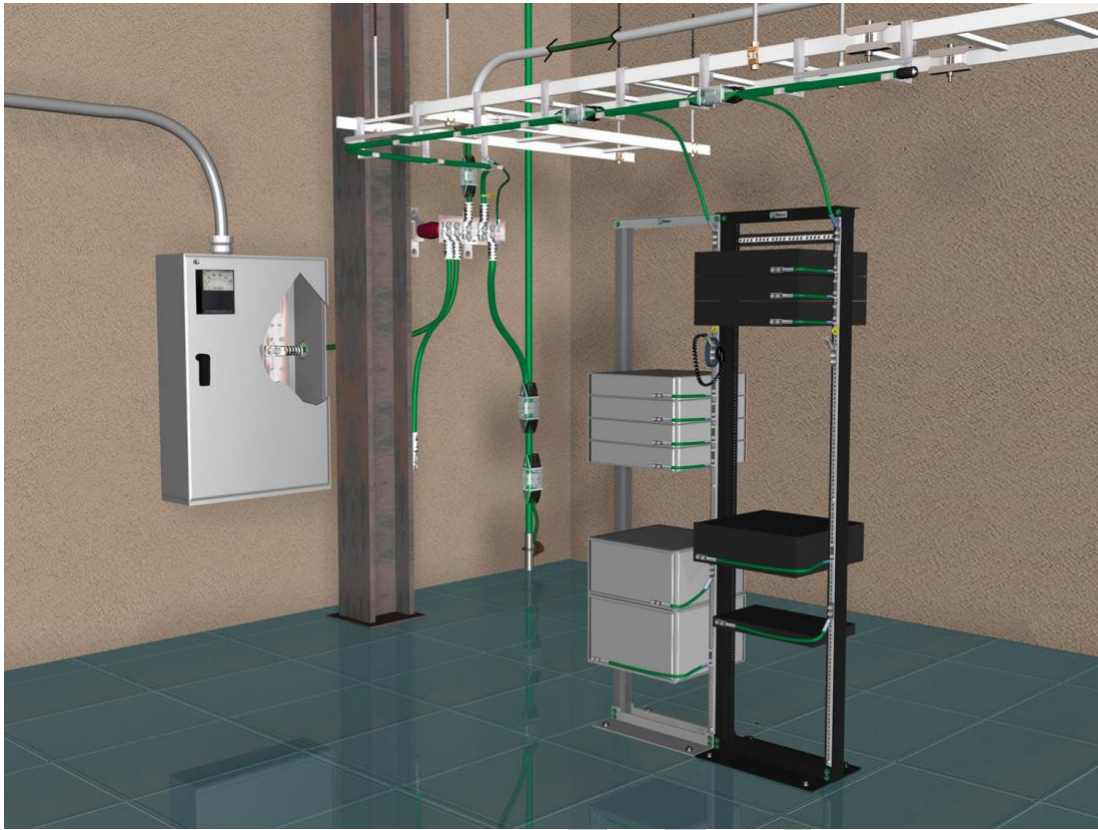
Figure 5: Grounding and Bonding in Telecommunications Room
