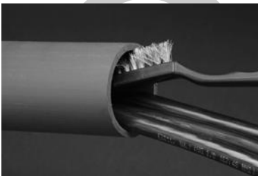
Clean conduit with wire brush.
